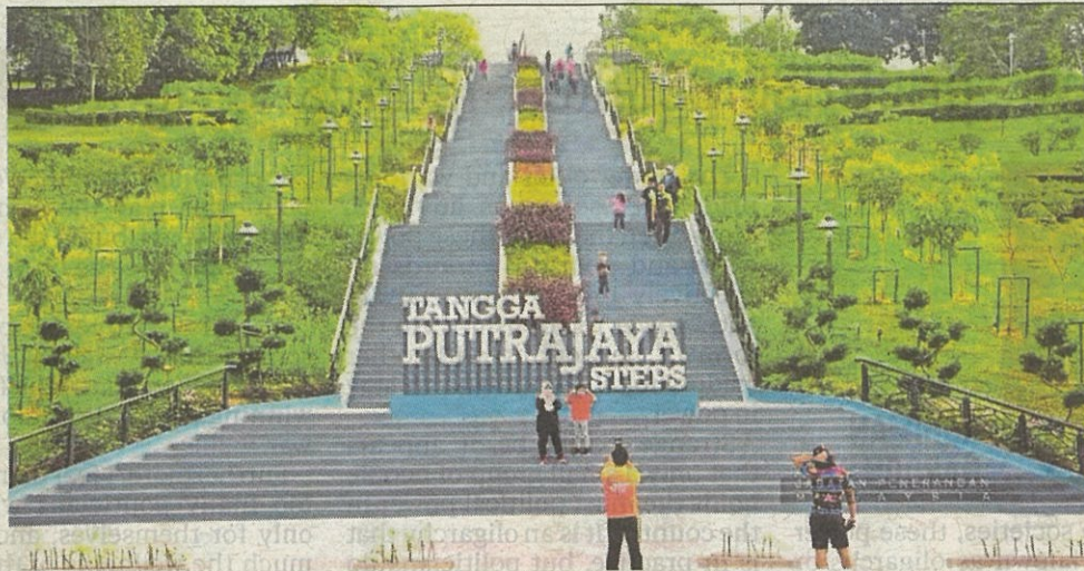
The Putrajaya Steps in Taman Putra Perdana in Presint 1, Putrajaya, has 250 steps with a climbing distance of 200m, and is 30m in height. FILE PIC
