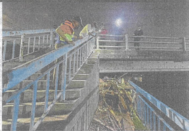
Mahadi (left) checking the situation at the Sungai Batu riverbank near Jalan Kasipillay, Kuala Lumpur.
