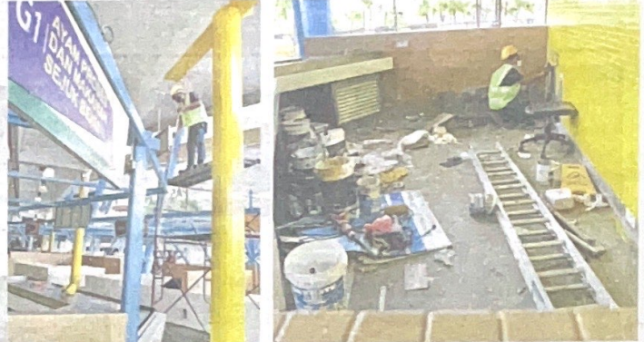
Upgrading works at the Precinct 8 market are on schedule.
